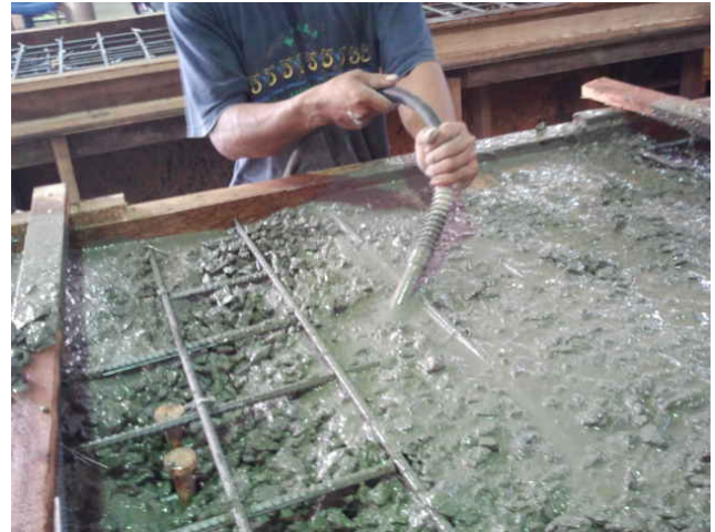
FIGURE 2. Compaction of concrete
