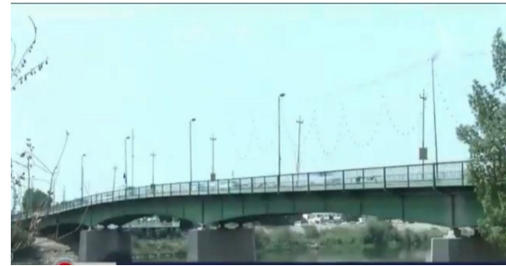
FIGURE 1. A general view of Al Kufa bridge
