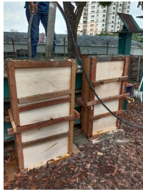
FIGURE 3. Casting of wall panel
