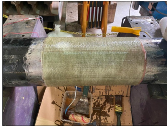
FIGURE 3. Application of composite wrap.
