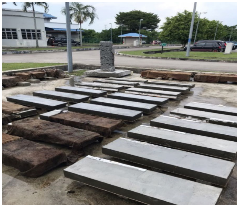
FIGURE 2. Curing process of wall panels
