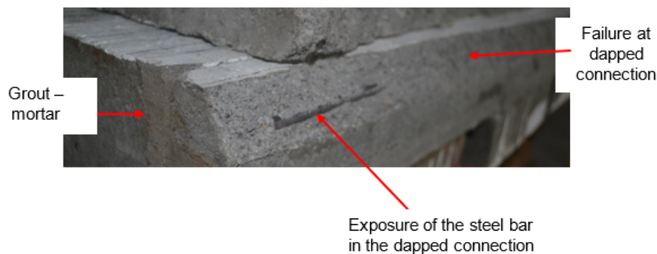
FIGURE 12. Failure of the wall connection at the joint interface of grout mortar and the dapped end for wall-to-wall connection Type 2
