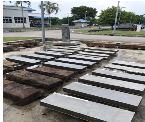
FIGURE 3. Curing of the wall panels
