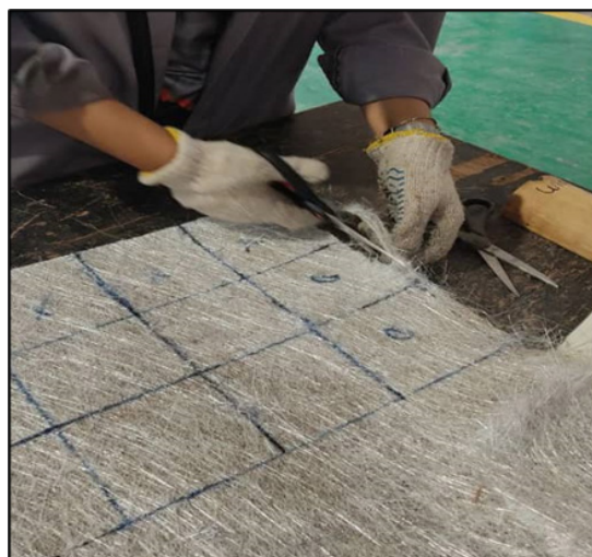
FIGURE 1. Preparation of GFRP sheet
