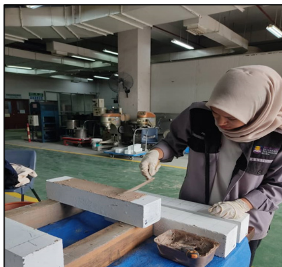
FIGURE 2. Applying the adhesive
